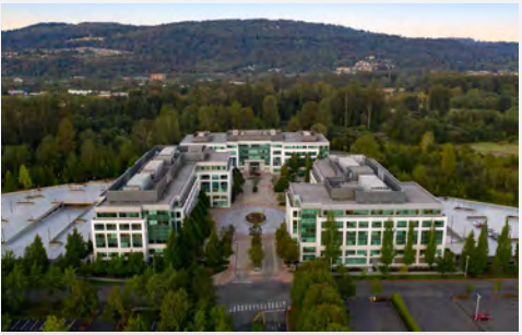
The ParQ I-90 CORRIDOR 411,279 RSF OFFICE SPACE AVAILABLE NOW
